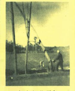
operates by hydraulic lift from a "stick" similar to an airplane, in the bucket. The man hoists himself about 30 ro 40 feet to top the tree.
